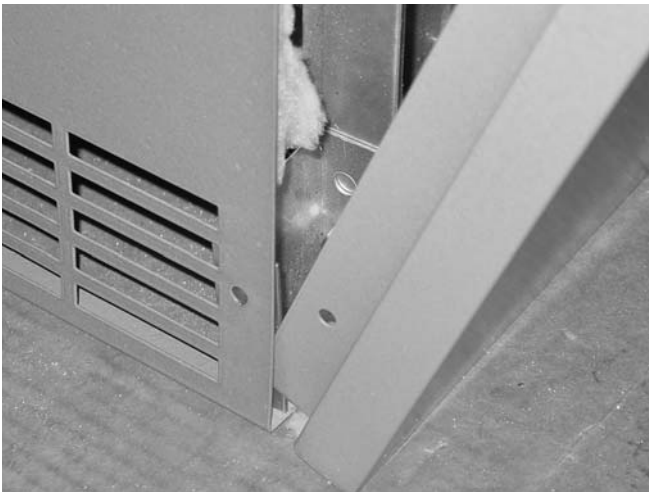
Figure 75 Jacket Side Panel Installation
