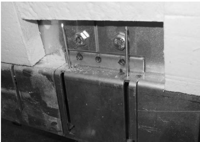
Figure 22A Burner Base Splice Insulation Boards
