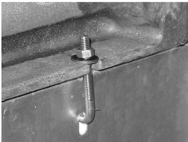
Figure 43 "J" Bolt Installation
