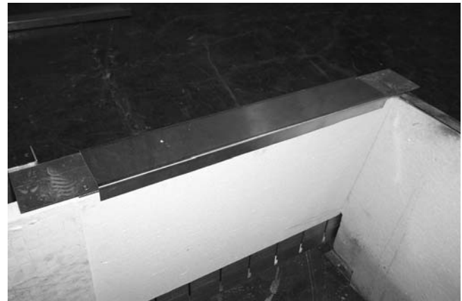
Figure 9B Refractory Retention Bracket
