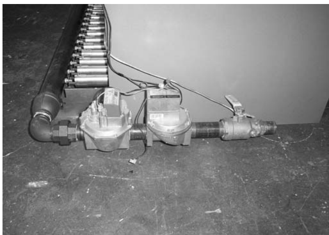
Figure 91 Gas Train, Valve Orientation
