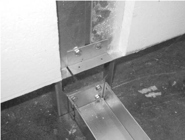
Figure 22A Burner Base Splice Insulation Boards
