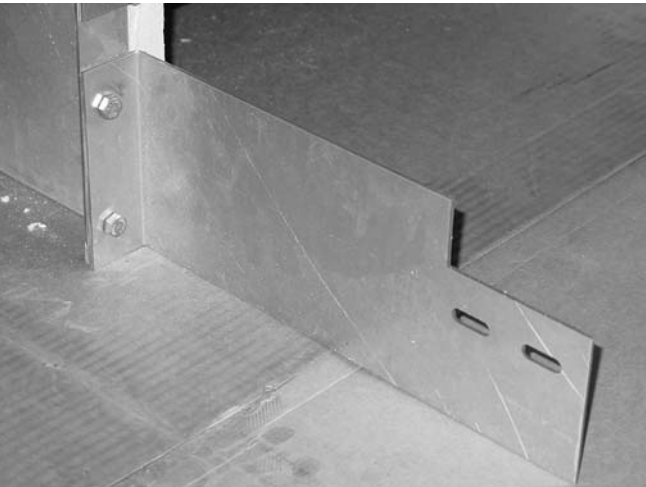
Figure 17 Manifold Bracket Attachment
