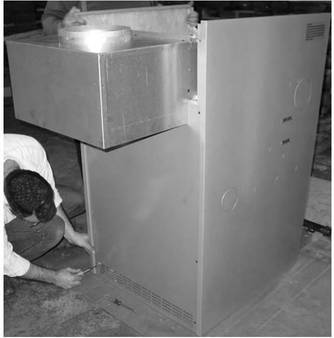
Figure 76 Jacket Side Panel Installation
