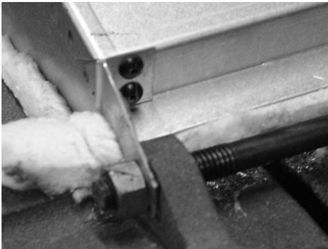
Figure 49 Flue Collector Bracket Installation
