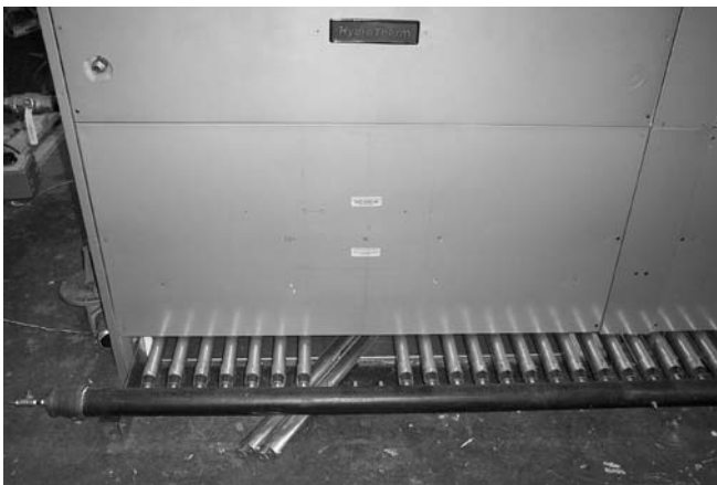
Figure 87 Front Access Panel 13 - 21 Sect
