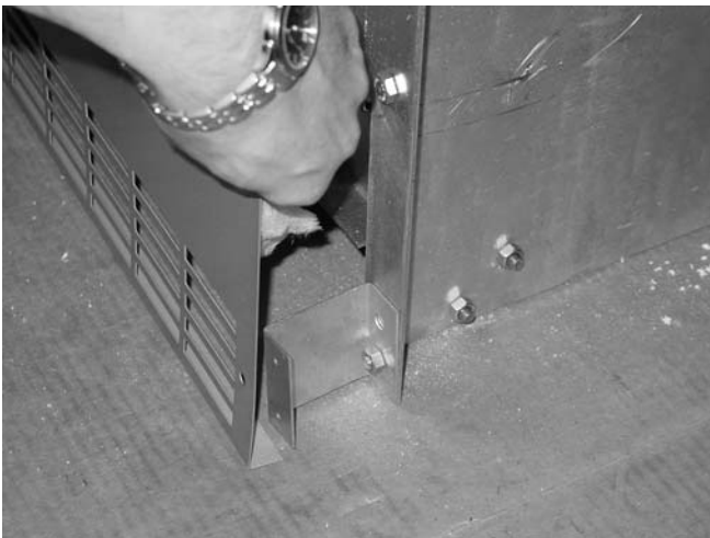
Figures 70 Rear Jacket Panel Installation Detail
