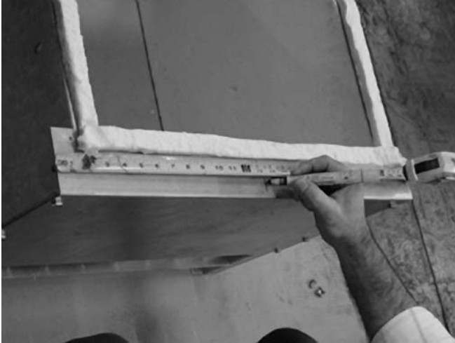
Figure 26B Marking Burner Base Rear Midpoint
