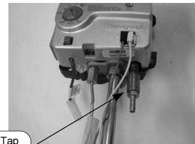
Pressure Tap Shown Installed
