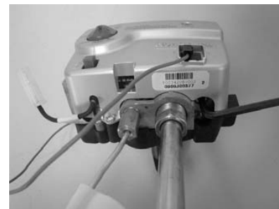
Gas Control shown in the "OFF" position
